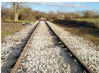
The track Extension - MSLR 2025
